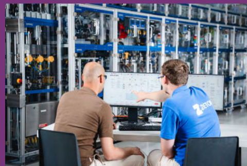
FAT of Continuous Manufacturing System (ContiUnity®)
