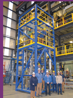
A petrochemical industry pilot plant
