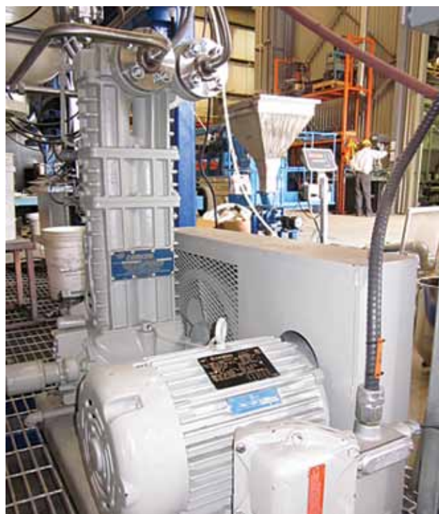
▲ Figure 1. An explosion-proof motor is used to run a compressor.
