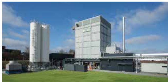
▲ Figure 4. A commercial-scale pyrolysis facility was constructed with modular equipment. Biomass-based pyrolysis is an example of the type of process that could benefit from locating small production facilities at geographically disperse locations, such as where there is abundant biomass.
