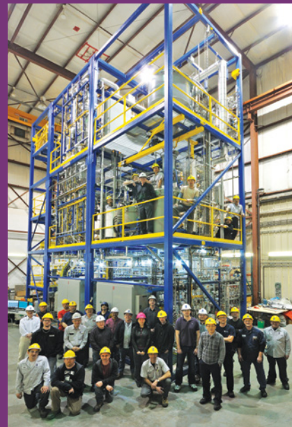
A biomass gasification pilot plant
