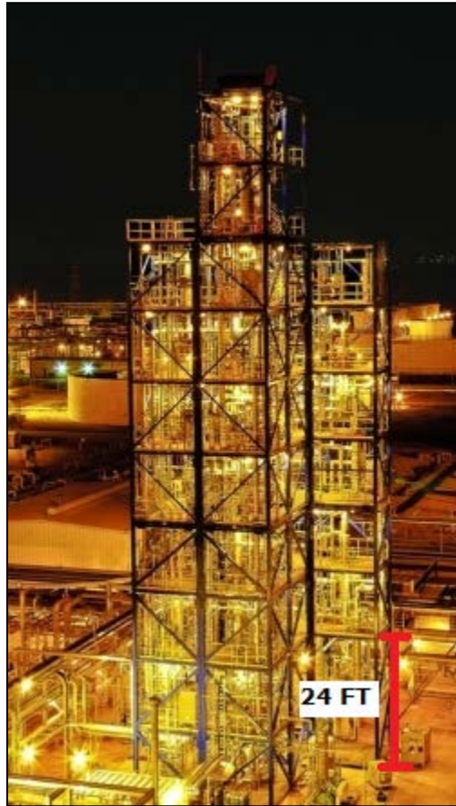
Figure 5. Ten-story pilot plant, only first two floors have pool fire as an applicable scenario.
